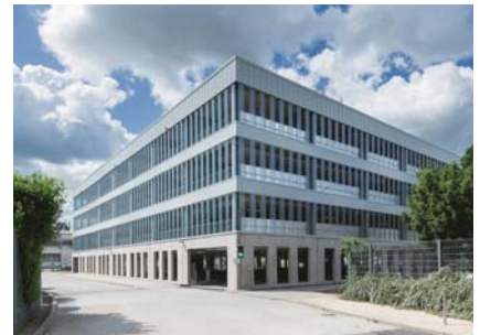
Multistory parking garages
