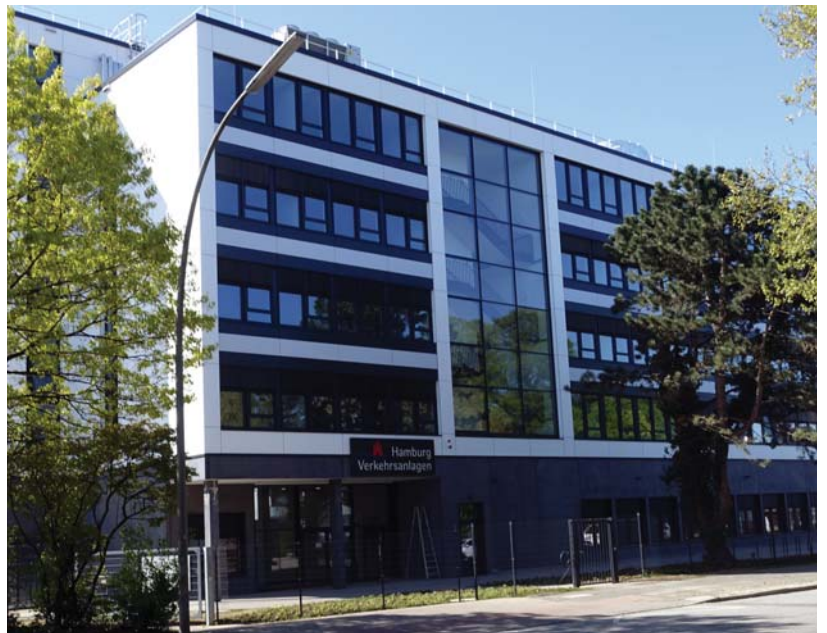
Smaller volume – office building, Hamburg, Germany
