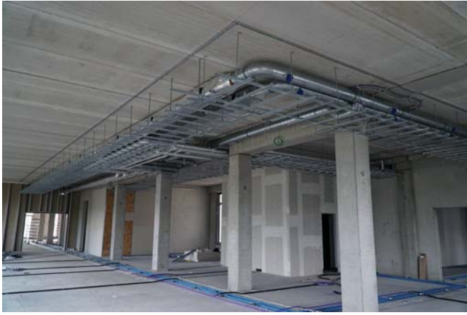
Lowering the structural ceiling height in selected sections for easier (collision-free) installation of suspended ceiling installations – Campus Loddenheide office building, Germany
