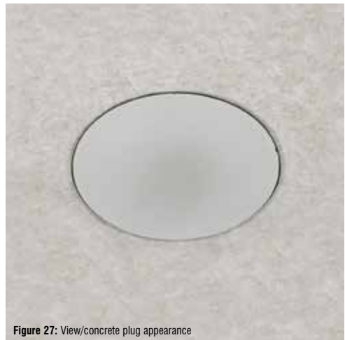
Figure 27: View/concrete plug appearance
