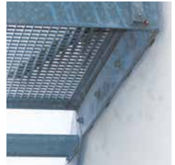
Stair fixing with DB anchors
