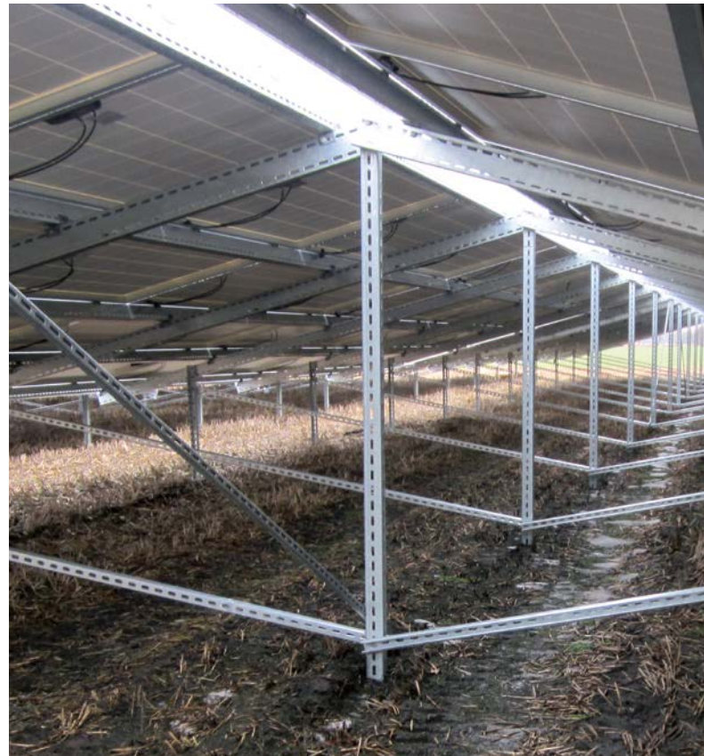
Module, Kristallin, 4-reihig, horizontal, Ost-West-Ausrichtung Modules, crystalline, 4-rows, landscape, east-west orientation
