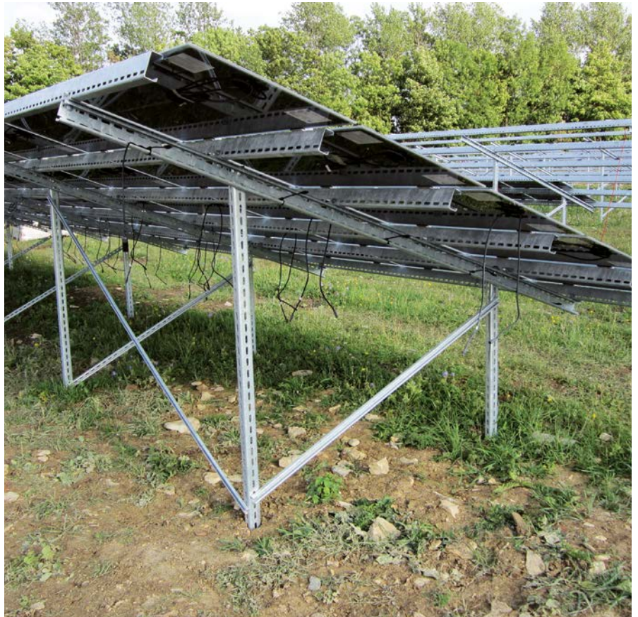
Module, Dünnschicht, First Solar, 5-reihig, horizontal Modules, thin-film, First Solar, 5-rows, landscape
