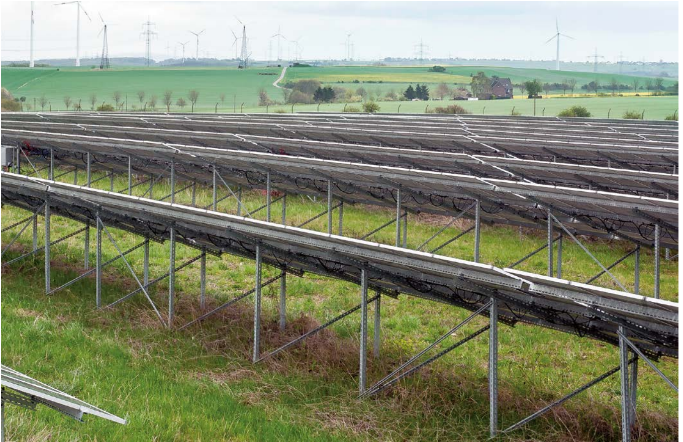
Module, Kristallin, 2-reihig, vertikal Modules, crystalline, 2-rows, portrait
