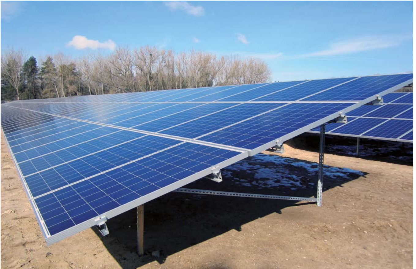
Module, Kristallin, 3-reihig, vertikal Modules, crystalline, 3-rows, portrait
