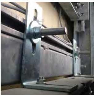
Fastening of lift doors in a lattice beam shaft
