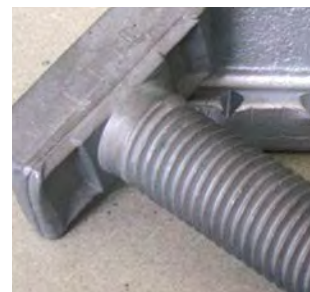
Notched teeth of the bolt press into the channel lip
