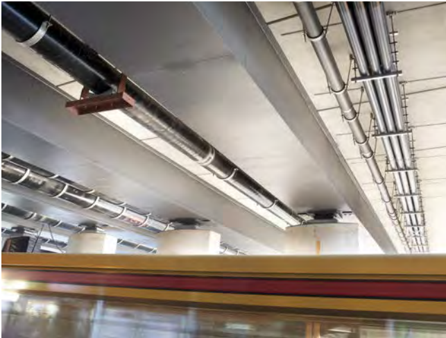
Spandauer Damm Bridge in Berlin, Germany
