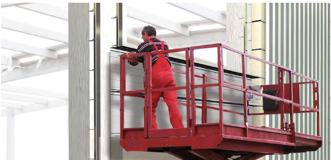
Installation of a multi-layer insulated profiled sheet metal wall.
