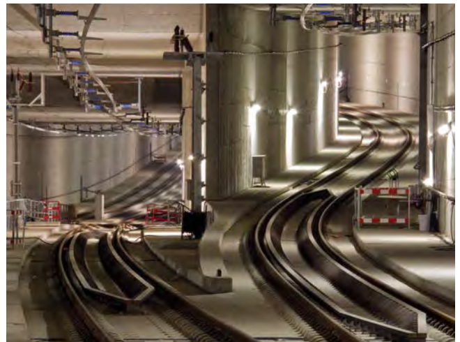
City Tunnel, Leipzig, Germany
