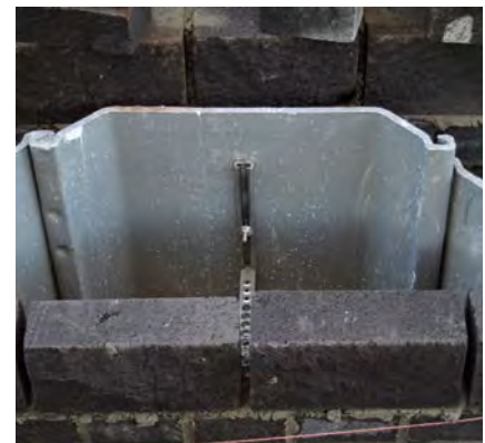
Connection of facing masonry to bulkhead wall
