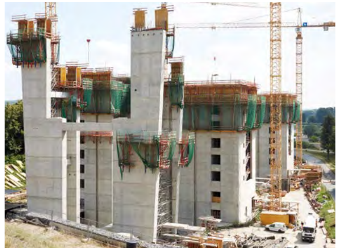
Niederfinow Boat Lift, Germany
