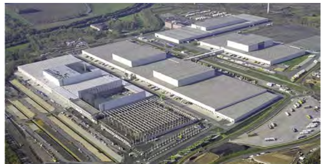
Attached on roof
