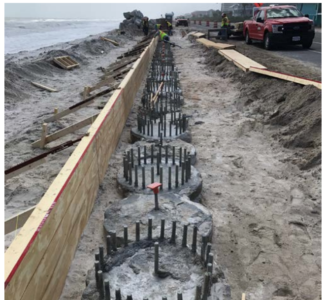
Coastal defence with 1,800 bored piles Flagler Beach, Florida, USA
