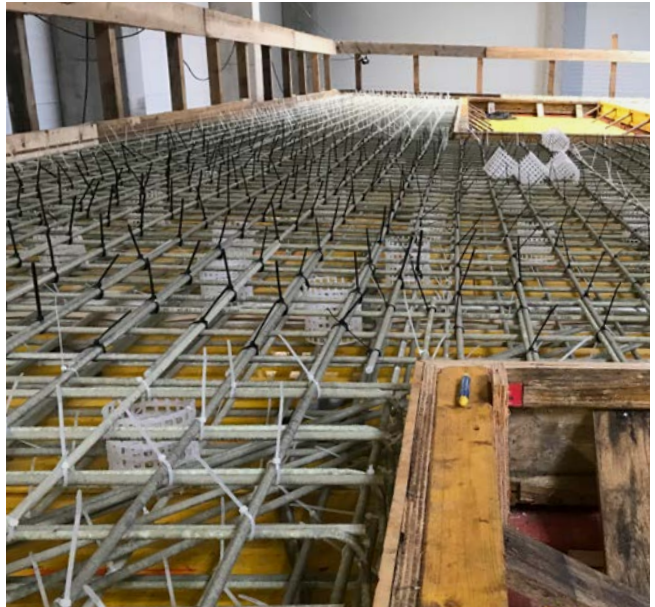
Ceiling slab reinforcement European XFEL GmbH, Schenefeld, Germany
