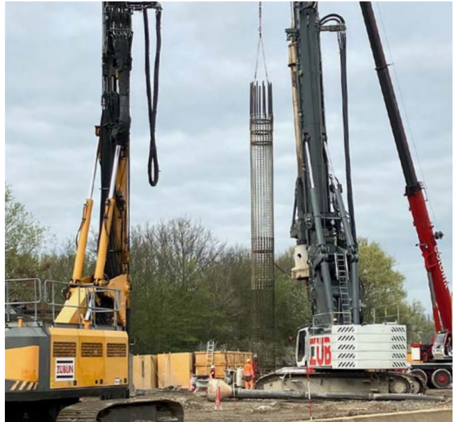
Bored pile- and diaphragm-wall reinforcement, Culvert-pipe "Rheindüker", Cologne, Germany
