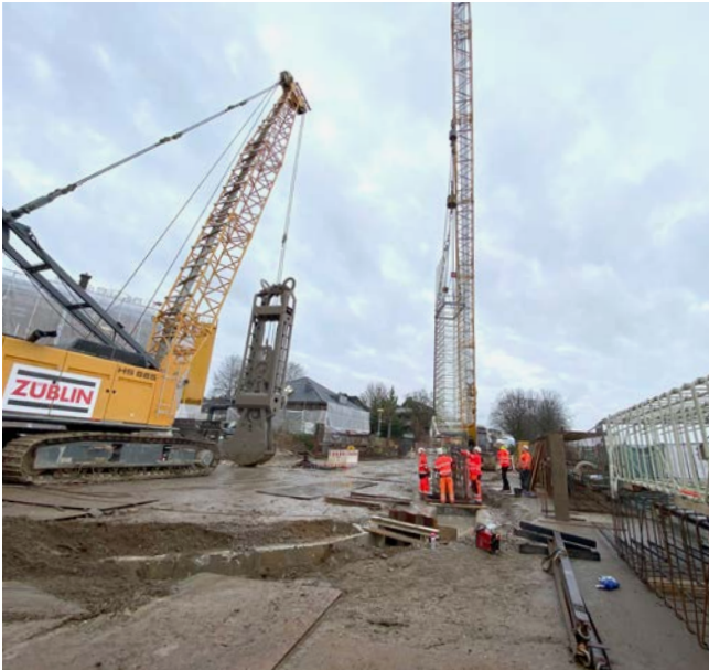
Bored pile- and diaphragm-wall reinforcement, Culvert-pipe "Rheindüker", Cologne, Germany
