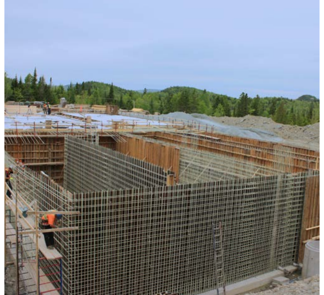
Tanks for sewage treatment plant, wall and floor slab reinforcement Thetford Mines, Québec, Canada
