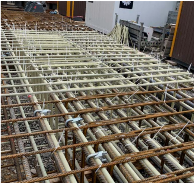
Diaphragm wall of motorway enclosure Schwamendingen, Switzerland
