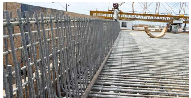
Installing FIBERNOX® V-ROD in bridge deck and concrete guard rails
