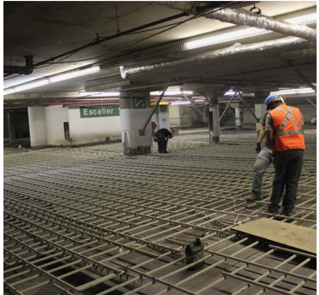
La Chancelière underground car park Québec City, Canada
