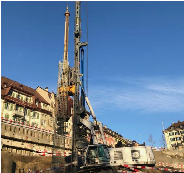
Bored piles in the Wildpark excavation pit Future train station, Bern, Switzerland
