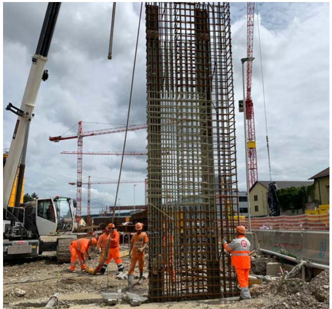
Diaphragm wall of motorway enclosure Schwamendingen, Switzerland
