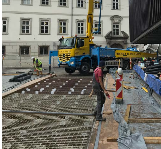
Creative concrete forecourt Haus der Musik, Innsbruck, Austria
