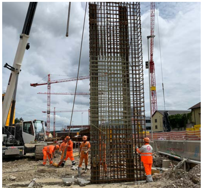
Diaphragm wall of motorway enclosure Schwamendingen, Switzerland
