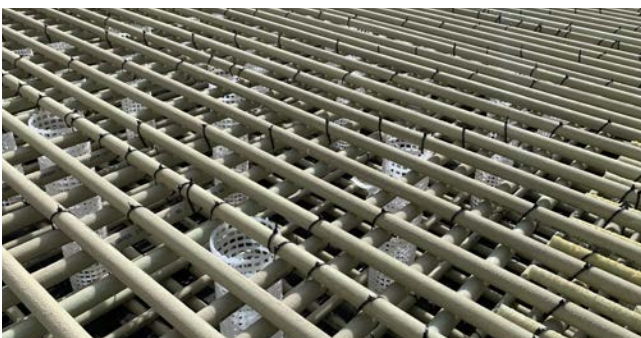
Floor slab of physics laboratory, University of Zurich-Irchel, Switzerland
